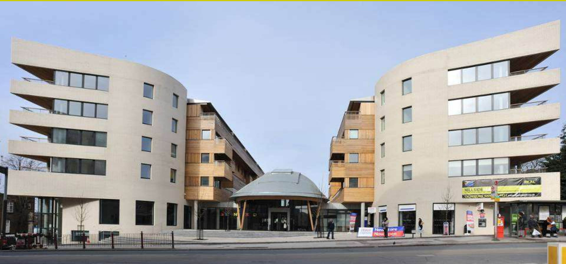
Stonebridge Hillside Hub HYDE HOUSING ASSOCIATION
