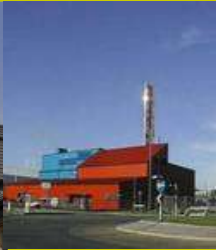
Southampton district heating with own CHP plant
